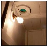
Other inside work includes a start on the wiring and testing of the lighting circuits and ducting many hundreds of feet of cables (pictures above). The illuminated bulbs are on test with a battery supply.
